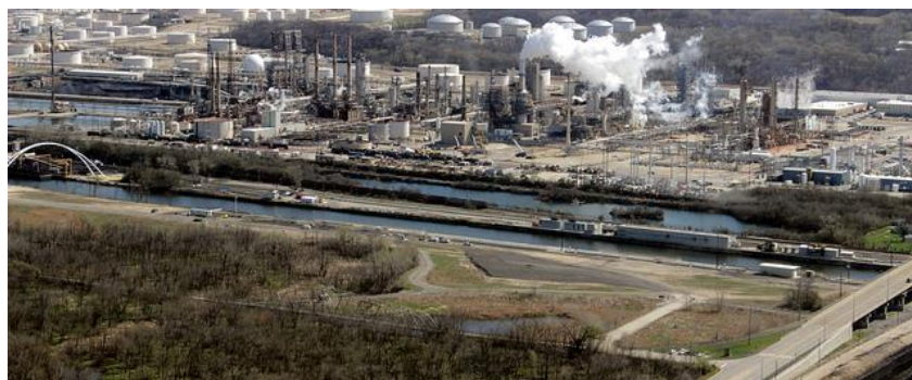
Aerial view of electric barriers project. Photo courtesy of USACE.
